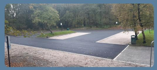
A new macadam surface on the lower car park was completed in October by a local company called The Asphalt Works. The scheme also included the laying of kerbs and drains and should make using the car park a more attractive option to visitors. Along with the village green drainage and footway improvements, this brings to a conclusion two of the largest projects the Parish Council has undertaken.
